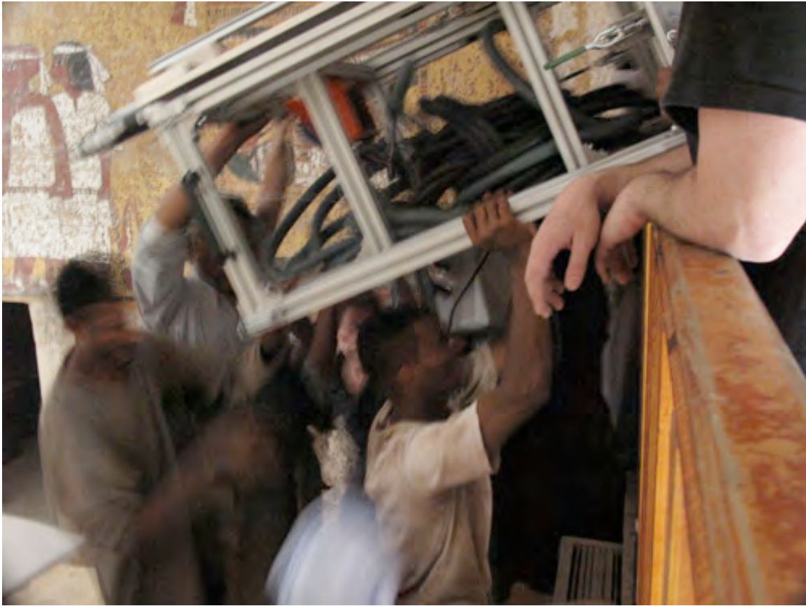
The Seti scanning frame being lifted into the tomb of Tutankhamun after the sarcophagus lid had been covered with a wooden structure to protect it during the work.
